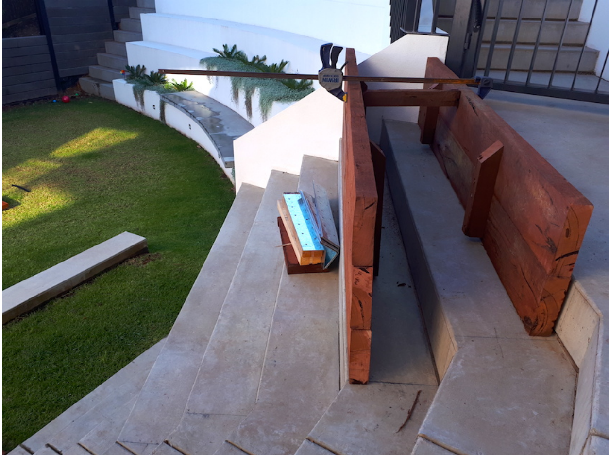
Two panels are in place, held together with a clamp. The tops of the panels are perfectly level.
