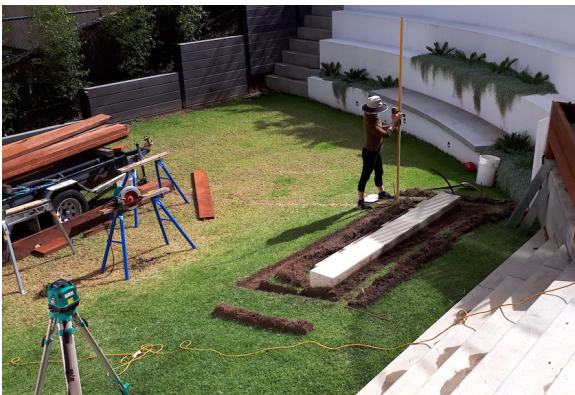
Sally recording measurements from the laser level to fine tune the exact depth of excavation needed for each side of the final garden bed.
